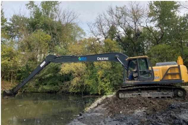
Photo 22. Mechanical sediment removal
