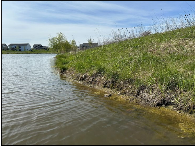
Photo 9. Moderate erosion exposing soil along the shore
