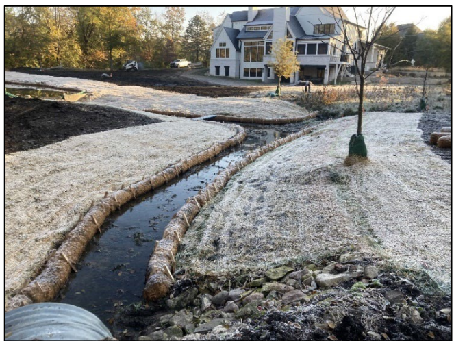
Photo 20. After – Stabilized with coir logs.
